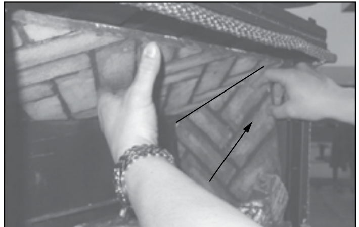
Figure 8.8 - Keeping the baffle elevated with your hand, put the right side brick into position. Rest the baffle on the right side brick.
